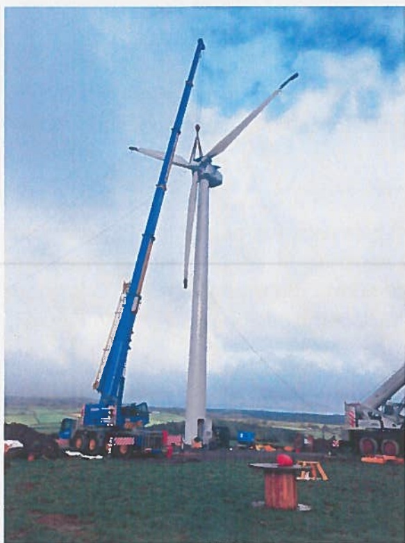
Figure 2 - Example 225kW Turbine in construction
